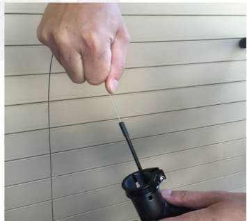
Pull cable through housing completely Pulling firmly at this point will eliminate any slack
